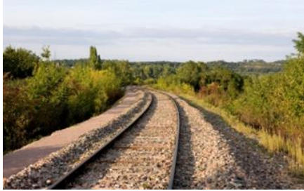
Cleaning and ecological maintenance line re-opening
